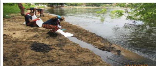
Clean up activities at the beach and magroves areas - deployment of absorbent boom
